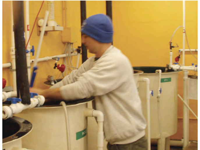
Figure 8. Cylindrical fiberglass tanks with sloped bottoms are used to hold planktonic larvae, which are transferred to other tanks by a siphon as illustrated.
