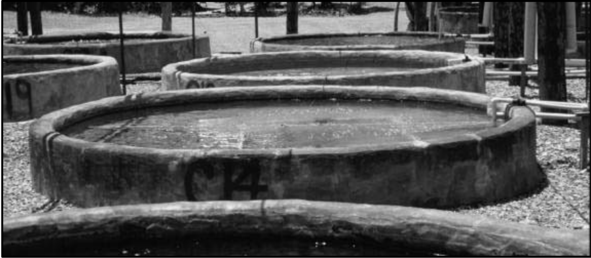
Figure 17. Round concrete tanks at ICLARM's Coastal Aquaculture Center on Guadalcanal, Solomon Islands.
