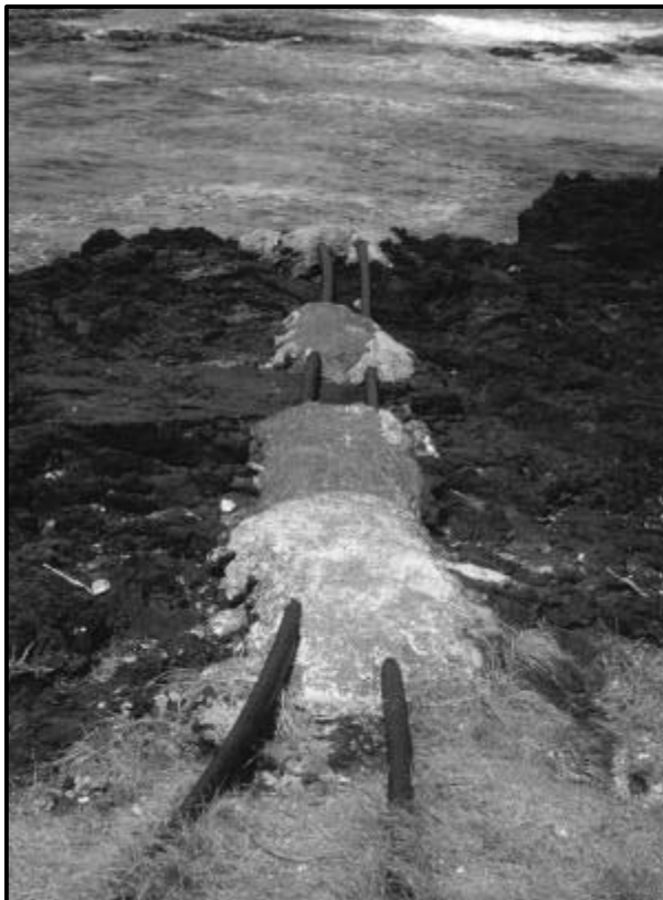
Figure 11. The need for clean, pollution free seawater sometimes means drastic measures. This seawater intake at the has been covered with concrete to protect it from the wave surae.
