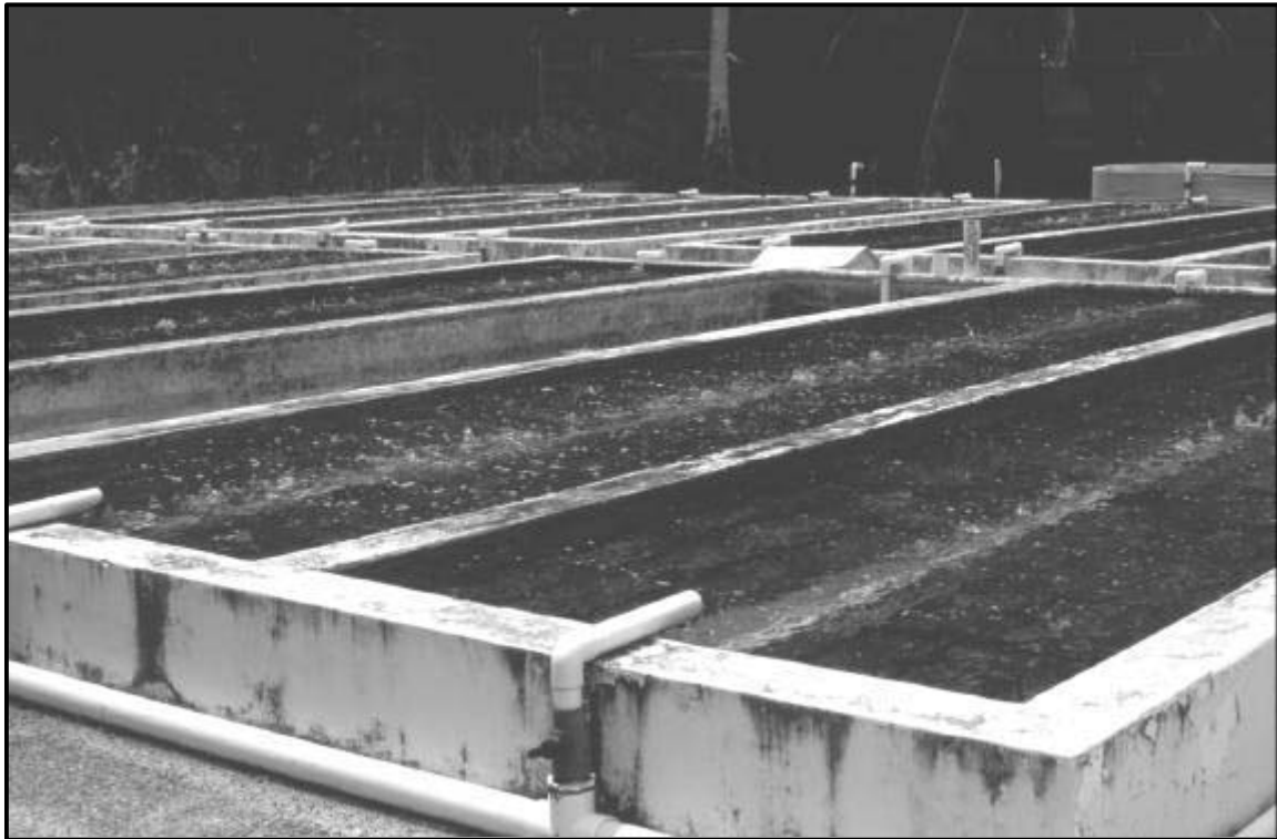
Figure 16. Rectangular concrete raceways at the Palau Mariculture Demonstration Center in the Republic of Belau.
